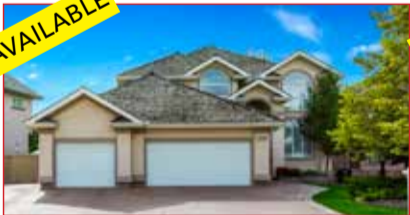
Twin Brooks $1,180,000 Beautifully renovated in Brookhollow. 4 bed, 3/12 bath. In floor heat walk-out basement. ML#E4448494
